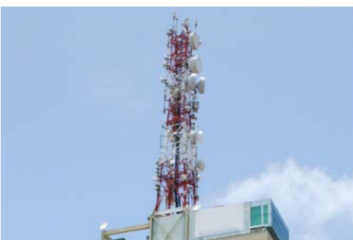
ROOF TOP TOWERS (RTT)
