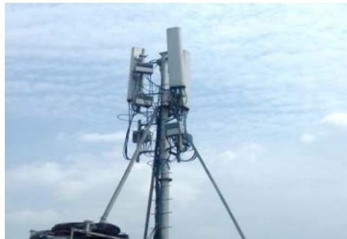
ROOF TOP POLES (RTP)
