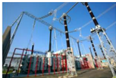
TBEA's 1000MVA/1000kV UHV AC transformer is used in the world's first commercial 1000kV Southeast Shanxi-Nanyang-Jingmen UHV Alternative Current Test Demonstration Project.
